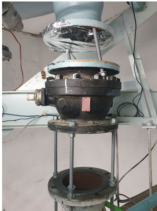
Figure 14 Old valve after asbestos gasket removal
