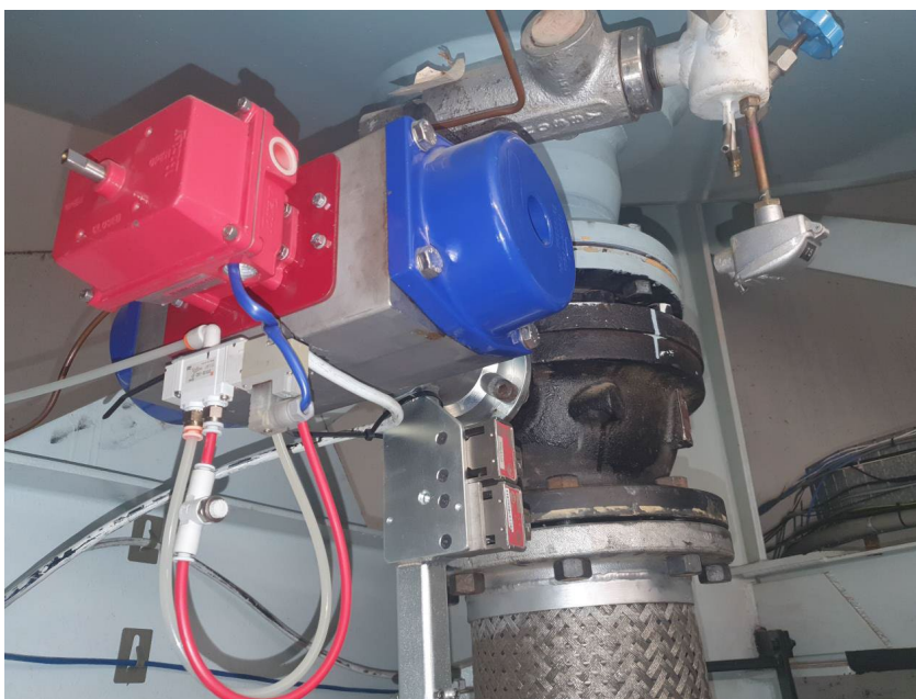
Figure 12 Old valve and bellows before removal
