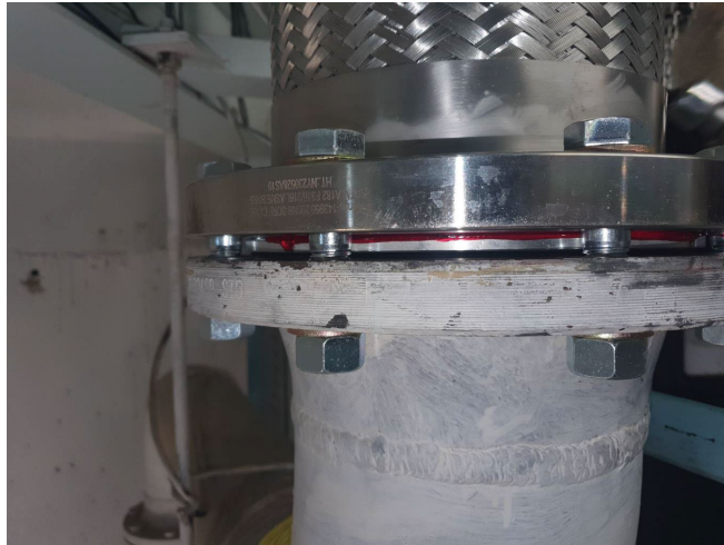
Figure 19 New bellows lower flange with Loctite 518 on both sides of al spacer disk
