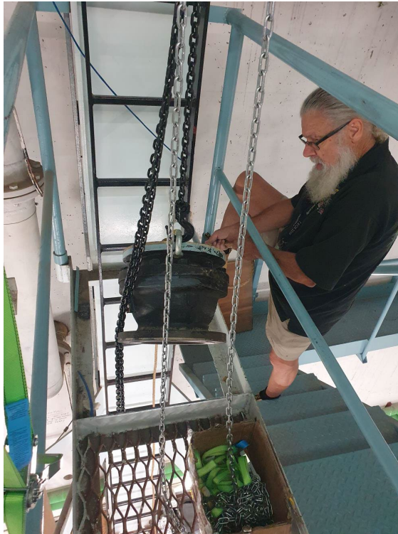
Figure 15 Using hoist to lower the old valve to ground level
