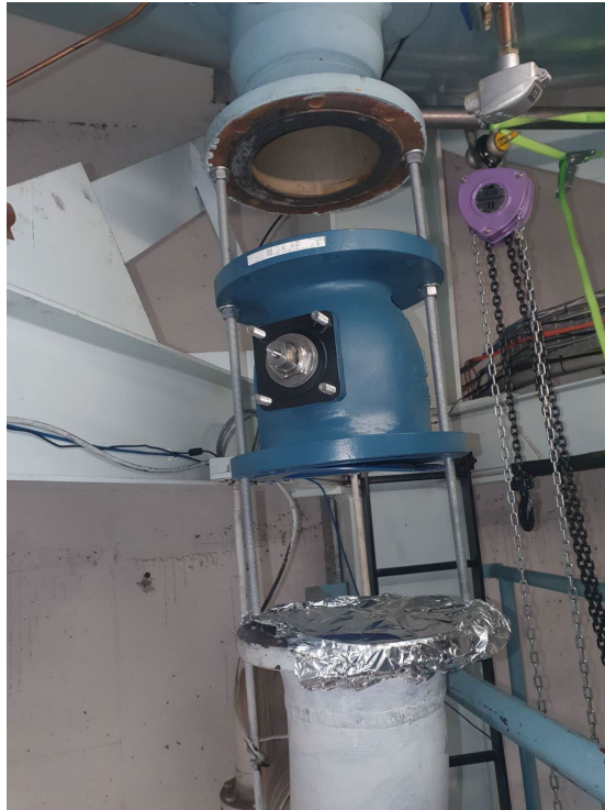
Figure 17 New valve lifted in place, final lift using threaded rods
