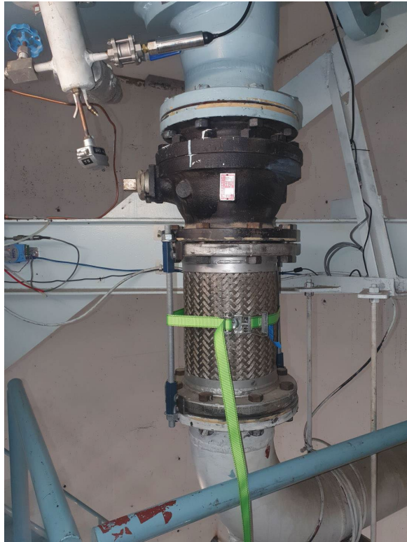
Figure 13 Threaded rods for squeezing bellows to allow removal
