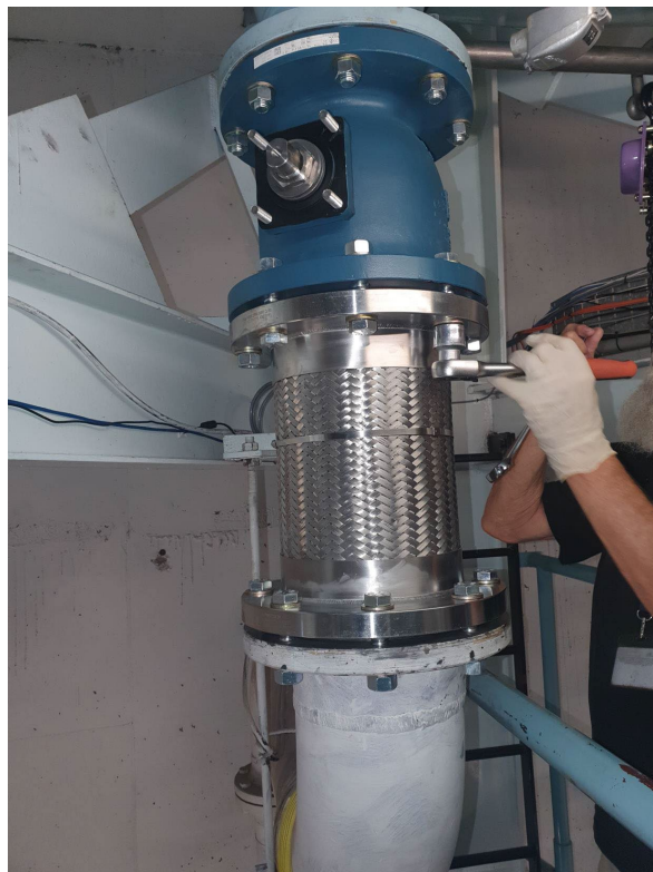
Figure 20 Final assembled new ball valve and bellows
