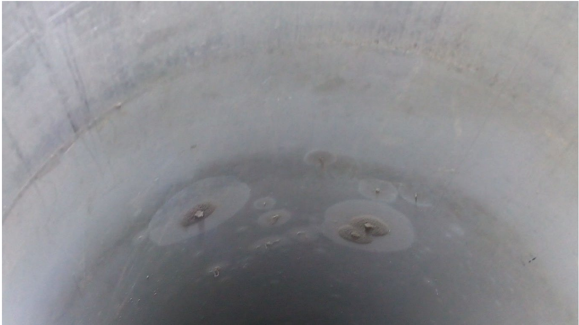
Figure 4 150kV beam focus cover “can” (air side) showing spark marks
