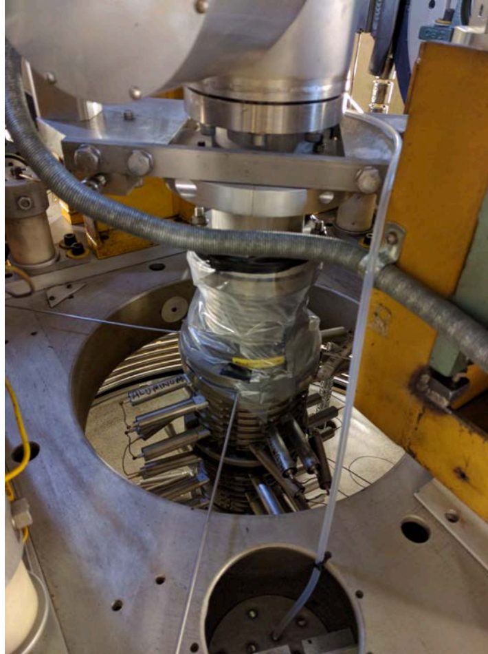
Figure 2 Terminal bellows in which a leak was found through the bottom flange
