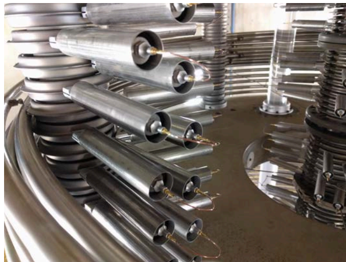
Figure 8 All post resistor leads in unit 4 were replaced with hardwire copper leads
