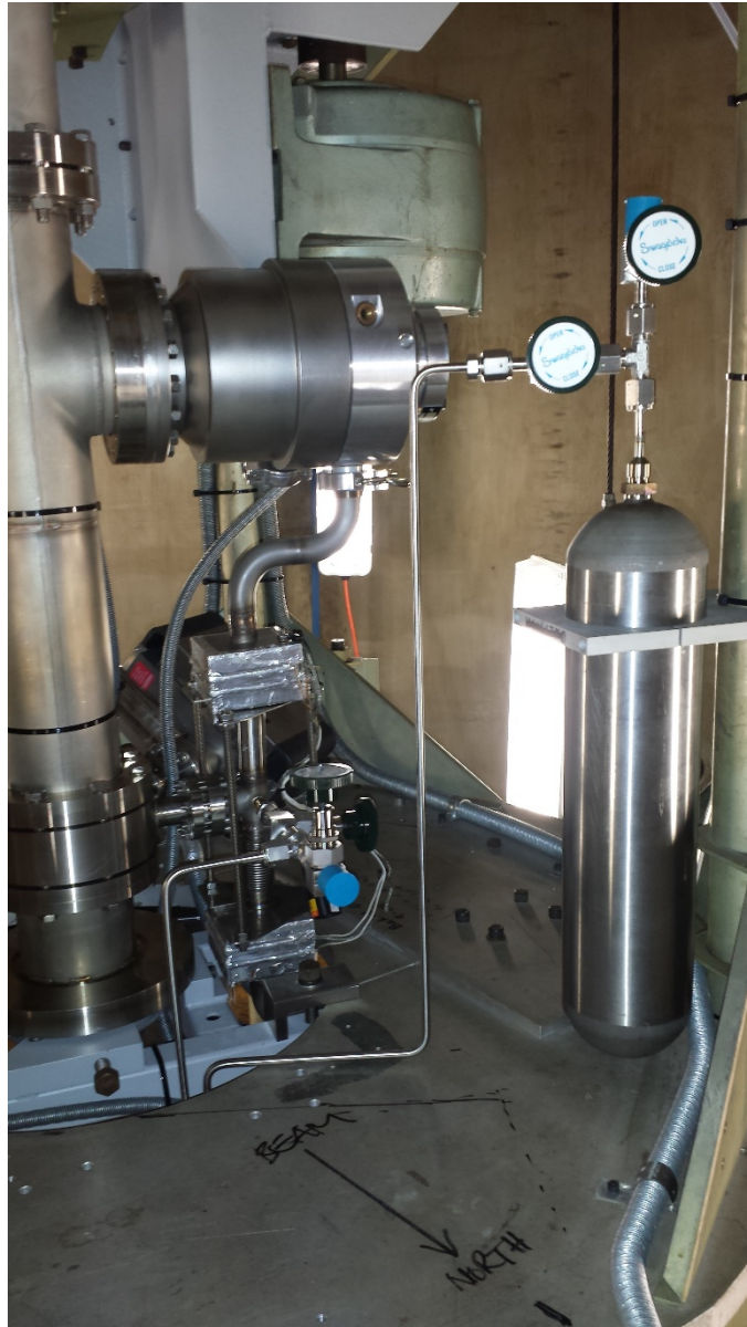
Figure 2 Gas stripper system with new VCR connections
