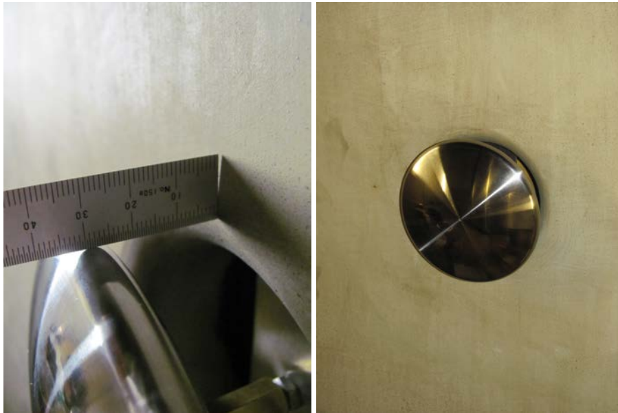
Figure 3 Stainless steel “mushroom” CPO electrode
