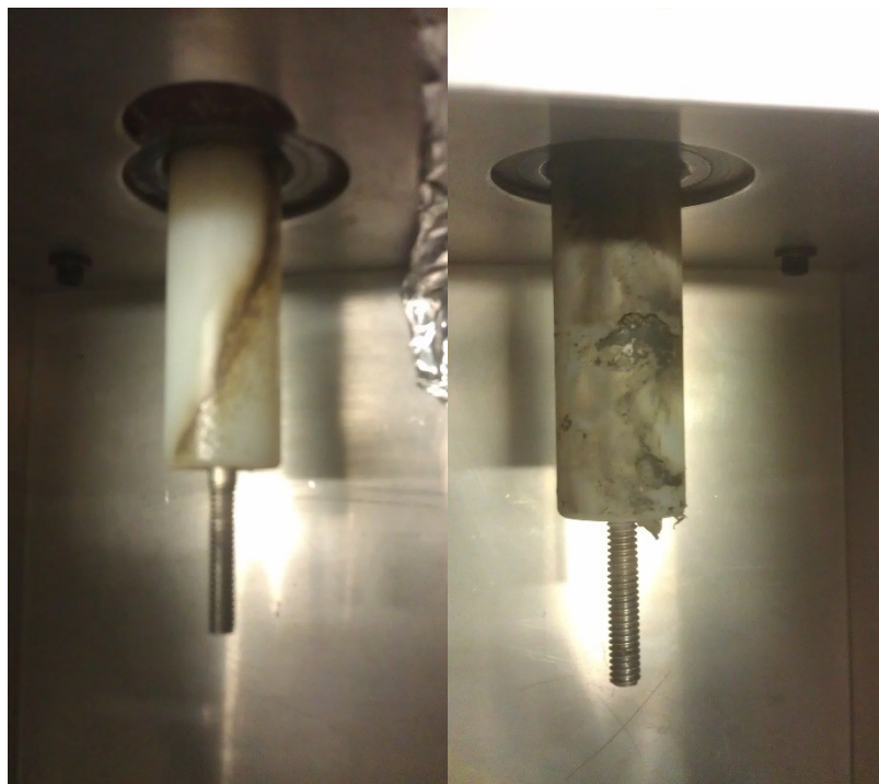
Figure 5 Damage to -ve (left) and +ve (right) charging system feed thrus
