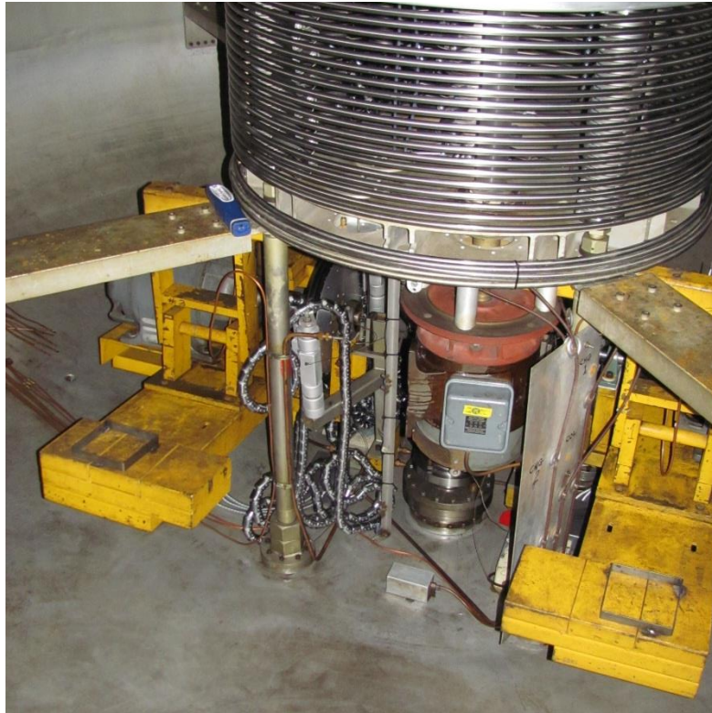
Figure 3 Location of broken chain #3
