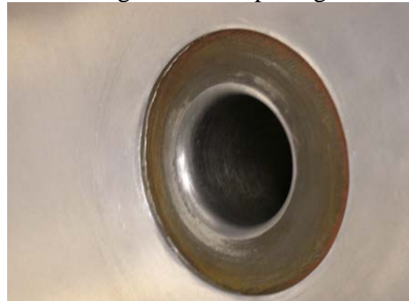
Refinishing done this opening.
